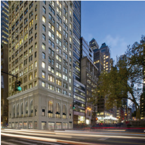
A rendering of the building after restoration Bohlin Cywinski Jackson
